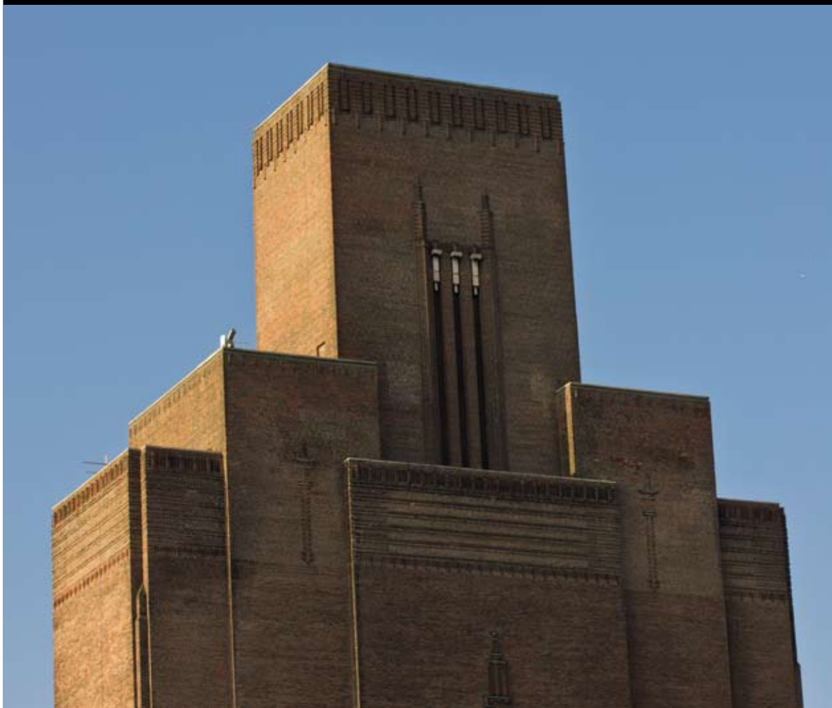
Woodside Ventilation Station
